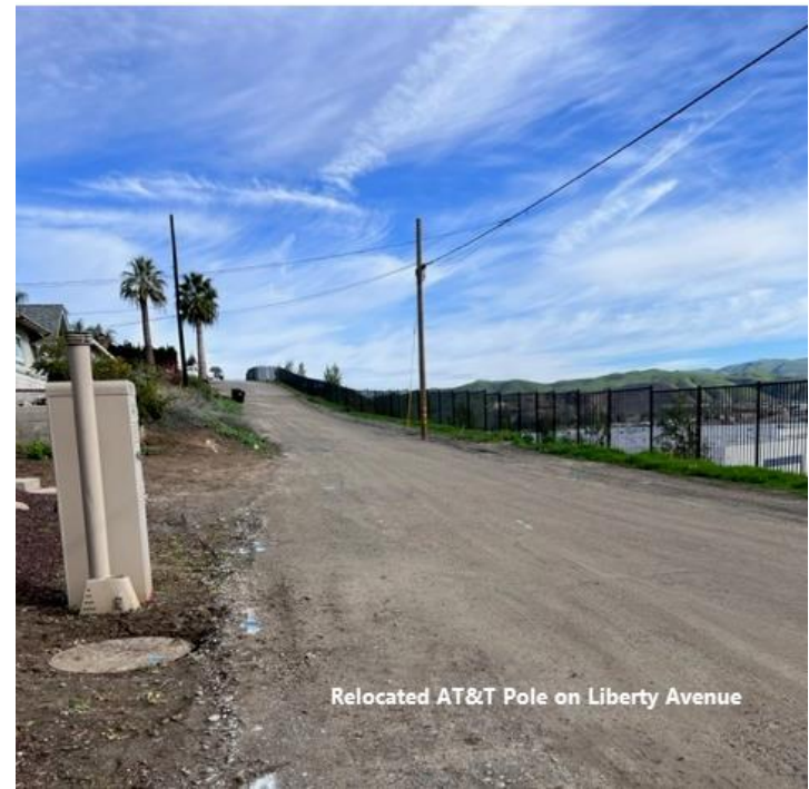
Relocated AT&T Pole Location
