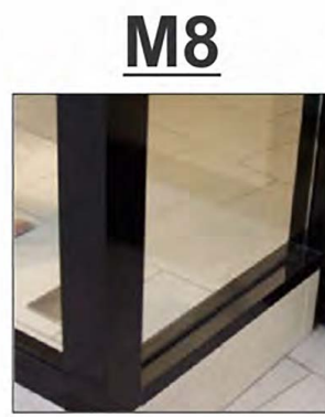
KAWNEER - ALUMINUM STOREFRONT SYSTEM FINISH: #40 BLACK ANODIZED AA-M10C21A44 / AAM45C22A44 ARCHITECTURAL CLASS
