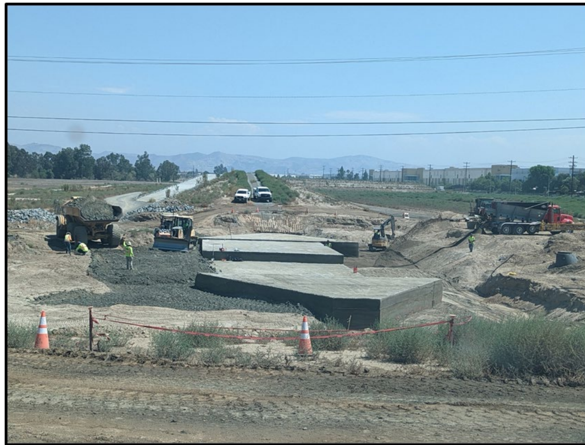
Foundation for utility protection, Auburndale Floodgate
