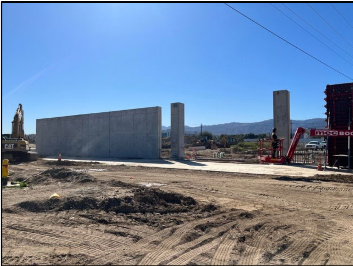
Auburndale Floodwall and Floodgate Columns
