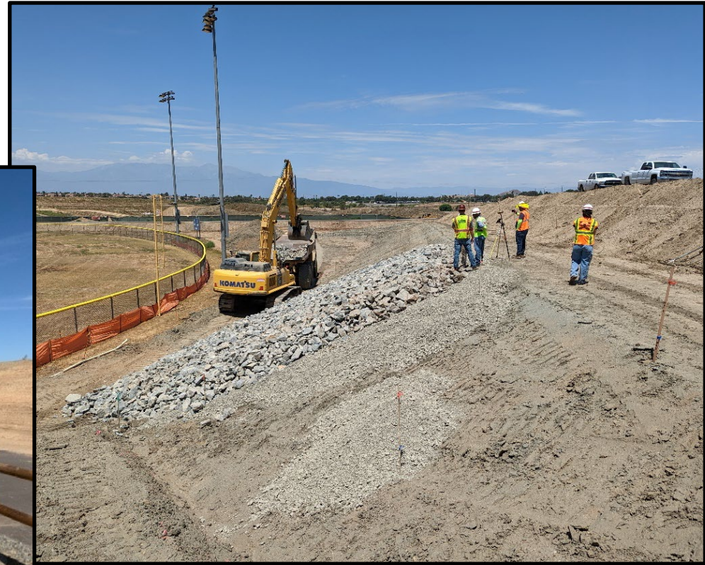
Placement of riprap (stone protection) in Butterfield Park section of Dike
