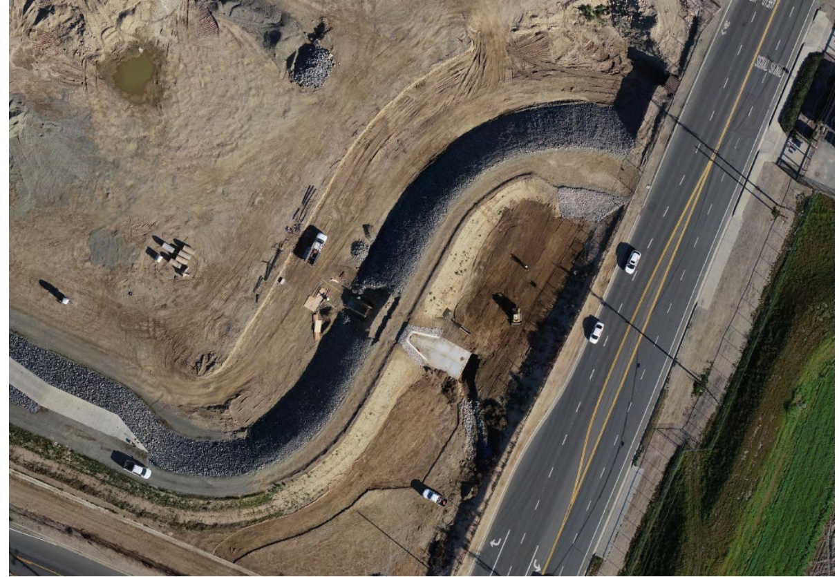
Dike tie-in at Lincoln
