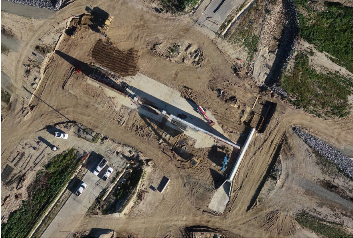
Floodwall site at Auburndale
