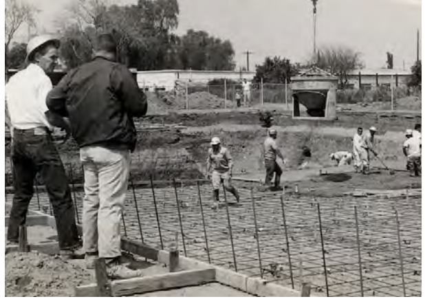
New swimming pool construction (c. 1967)
