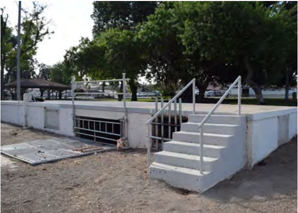
Former Pump Building
