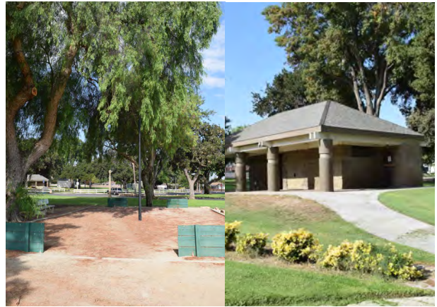
Horseshoe Pits / Restroom Building
