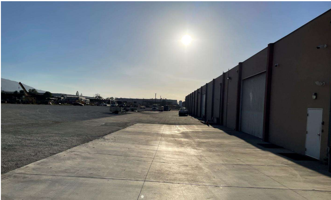
Photo 5: Side of Building, facing West
