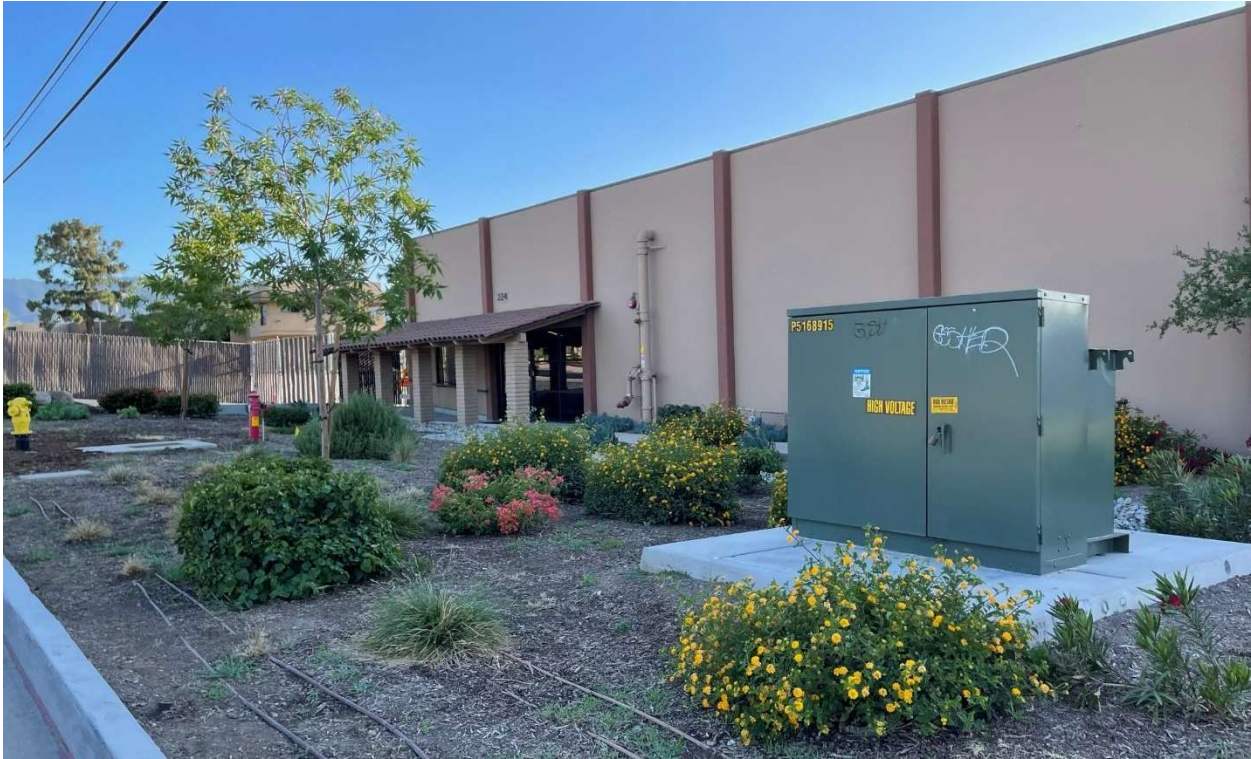
Photo 4: Front Building Façade
