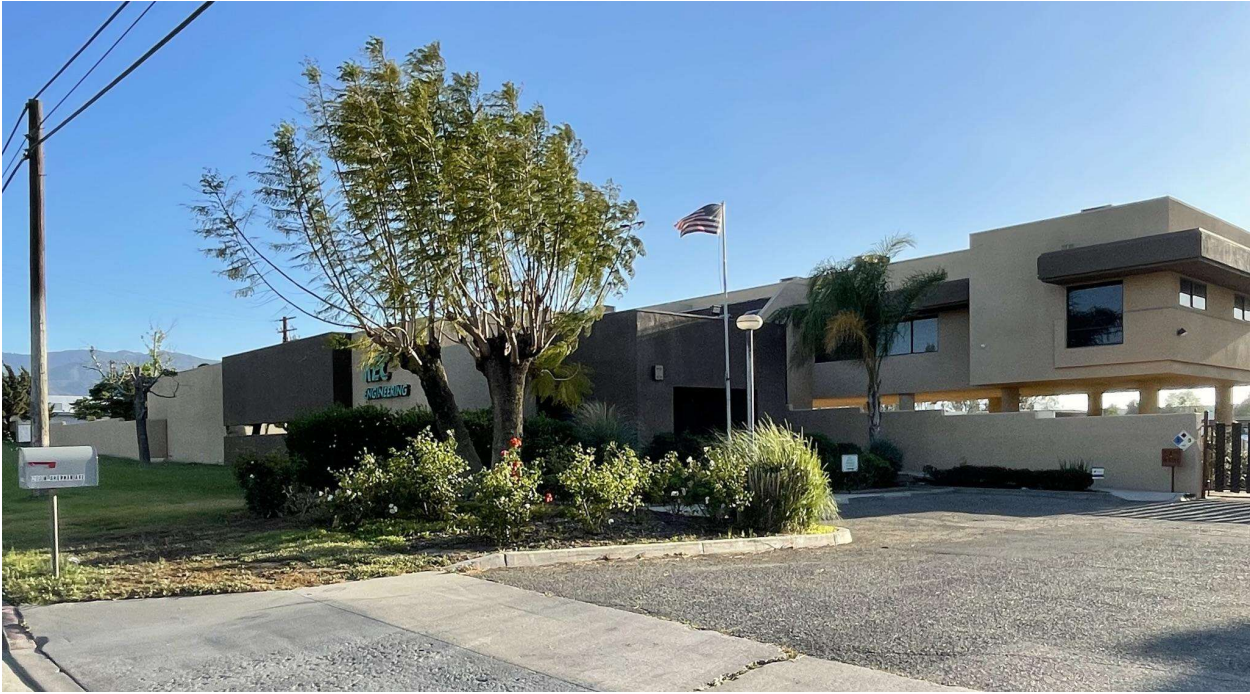
Photo 8: N. Sherman Ave, Facing front façade of 200 N Sherman Ave
