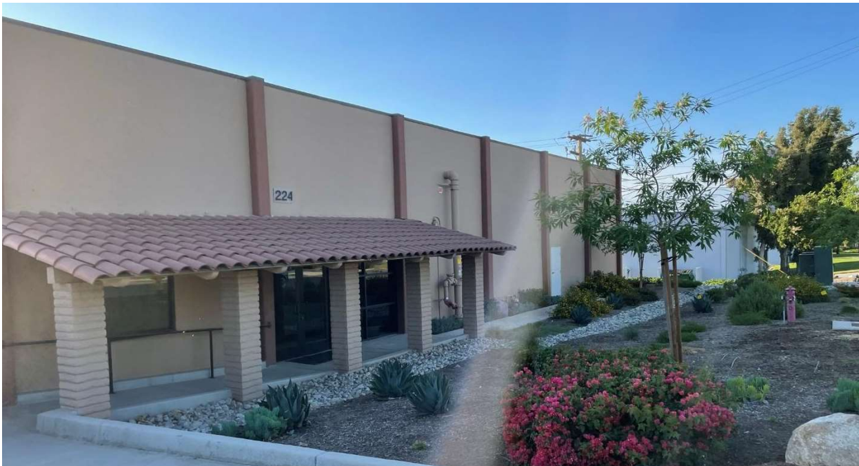
Photo 1: Front Building Façade
