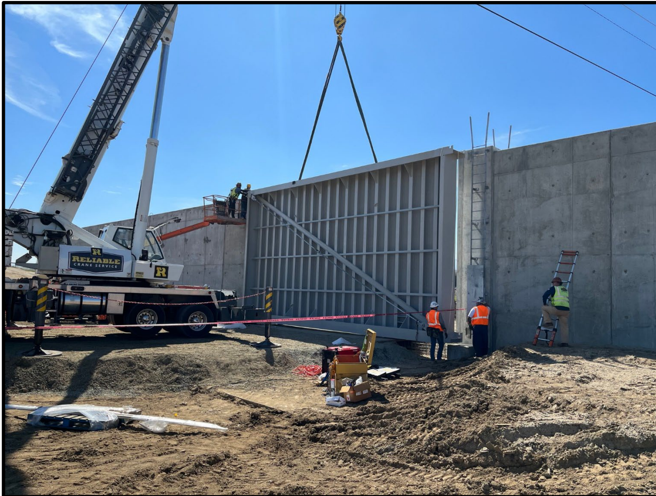
Floodgate Installation from March 2023
