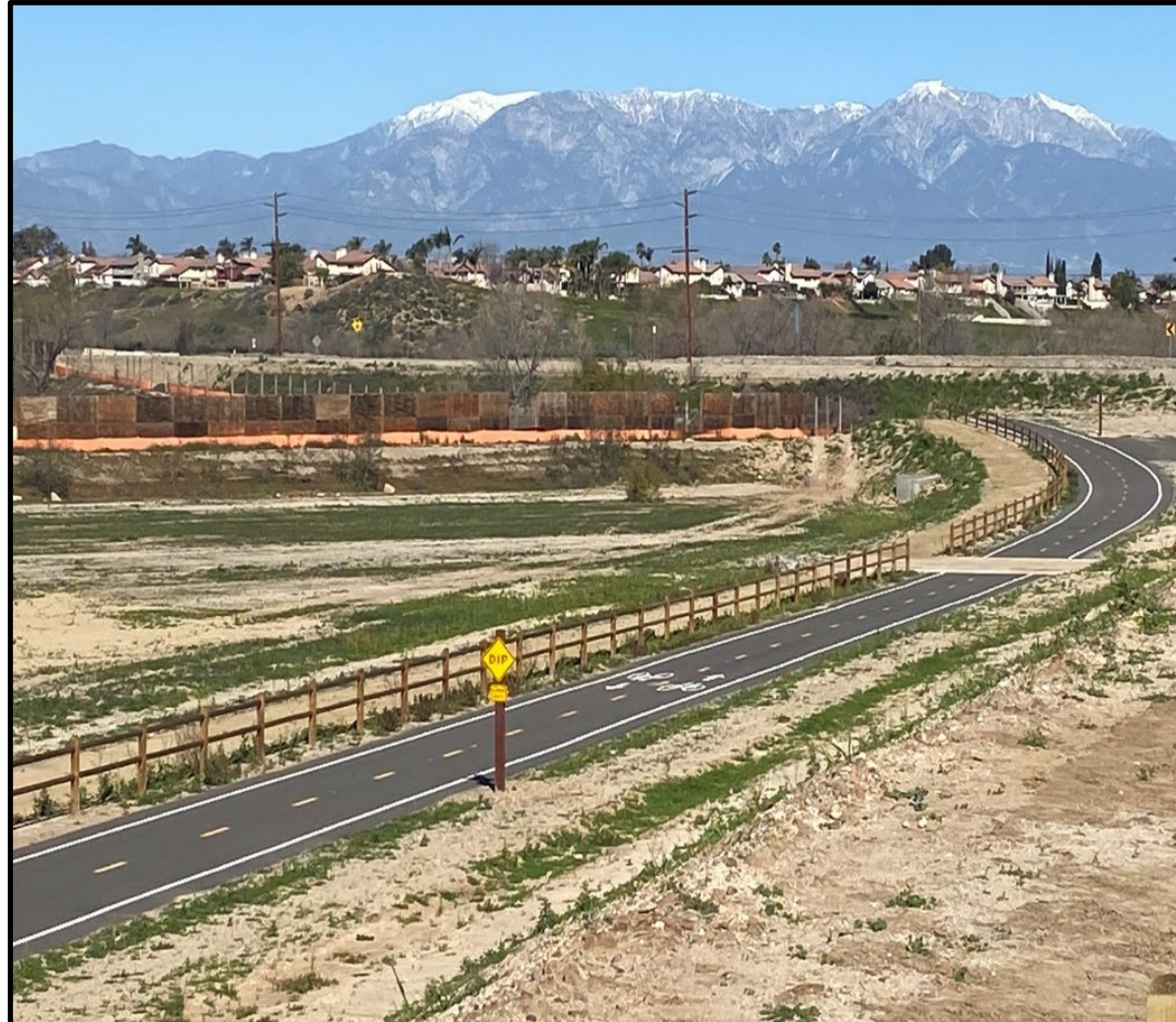
New bike path along the adjacent Santa Ana River Trail (Phase 4)
