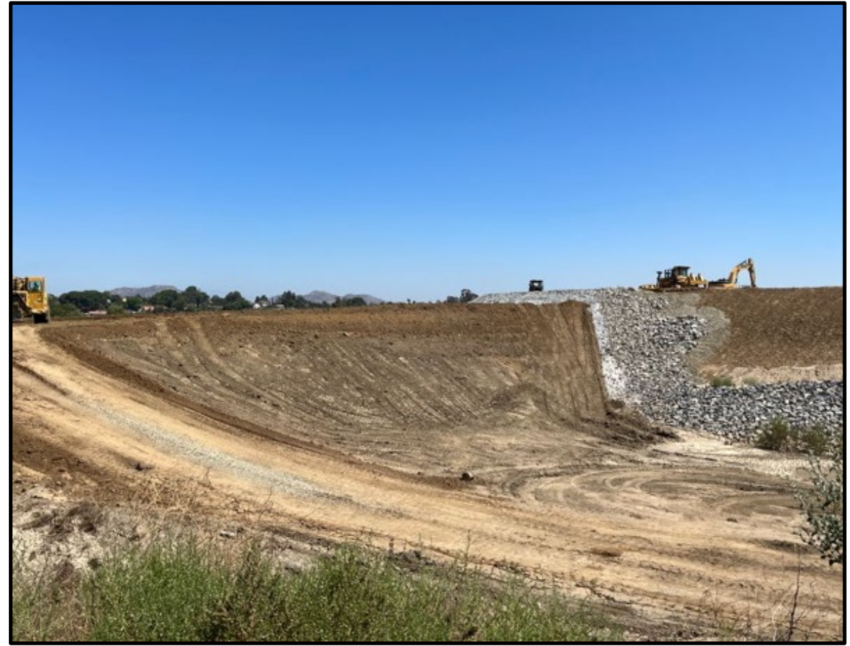
Backfill and riprap replacement along Rincon Street and Dike
