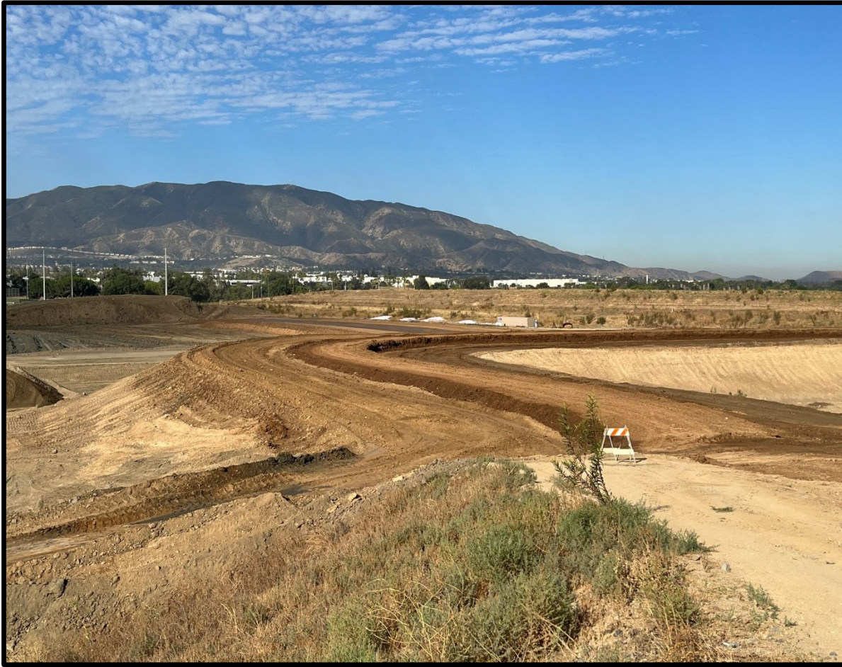
New Rincon Dike near future Rincon Street alignment
