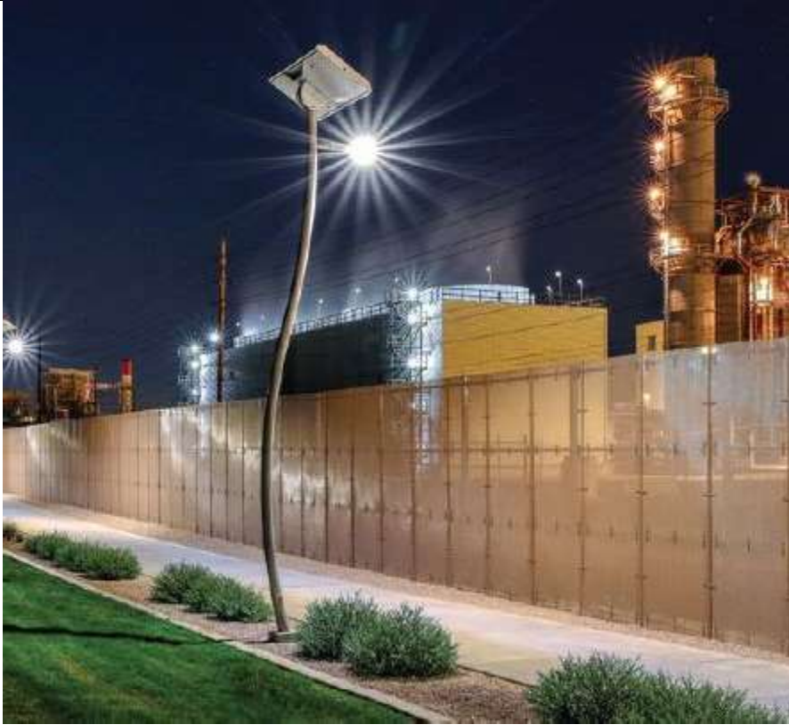
Figure 3: Typical Solar Lighting-Sample
