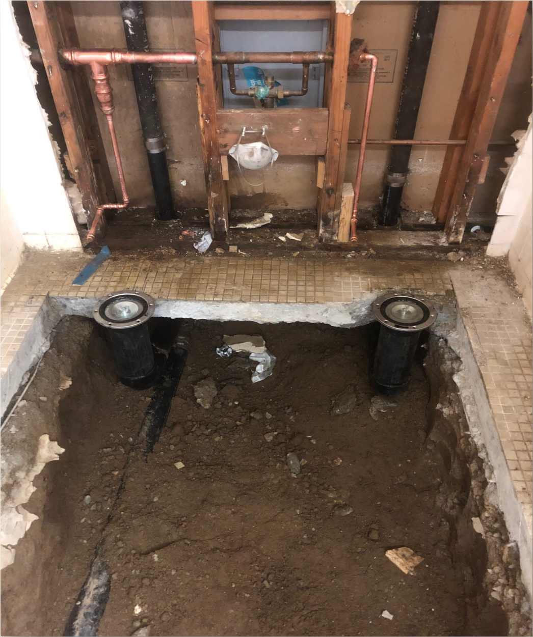
New ABS Plumbing Installed:
