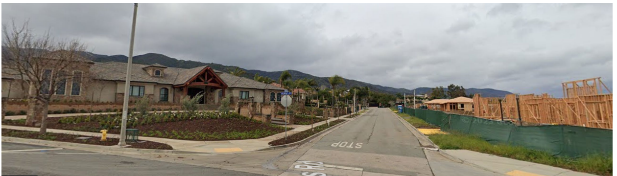
Romans Road looking toward the West
