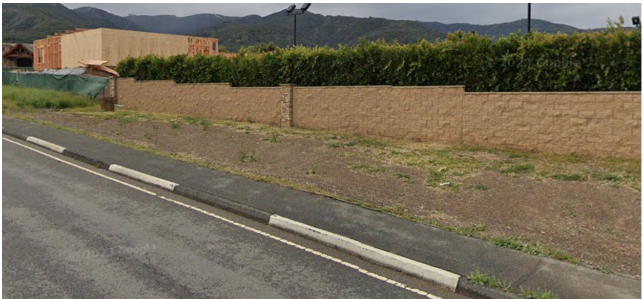
Existing block wall along Gilbert Avenue to continue with Variance
