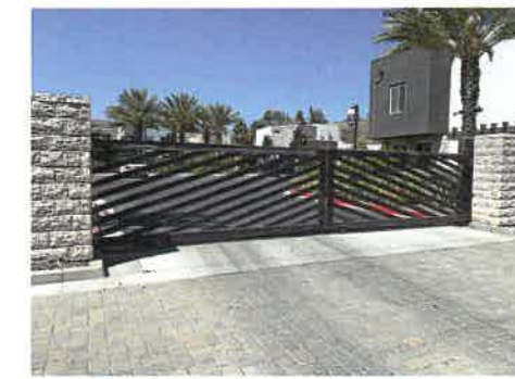
EXISTING TUBULAR STEEL VEHICULAR SLIDING GATE
