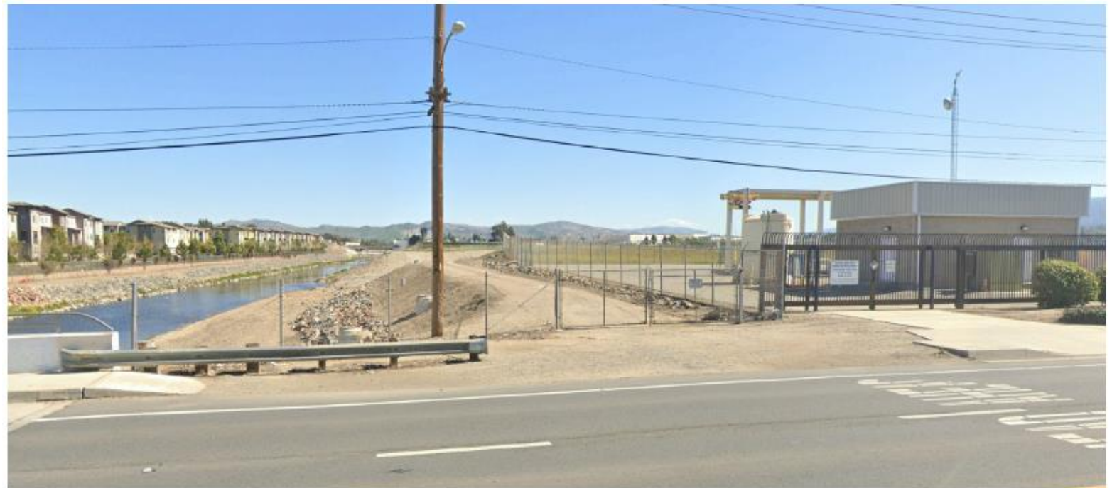
The Public Safety Way trail connects Lincoln Avenue to North Cota Street via flood control channel.
