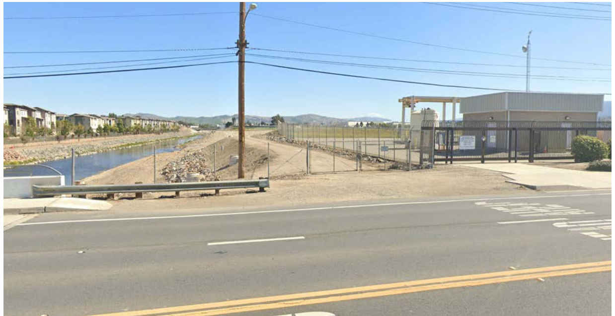
The top ranked Public Safety Way trail connects Lincoln Avenue to North Cota Street via a flood control channel
