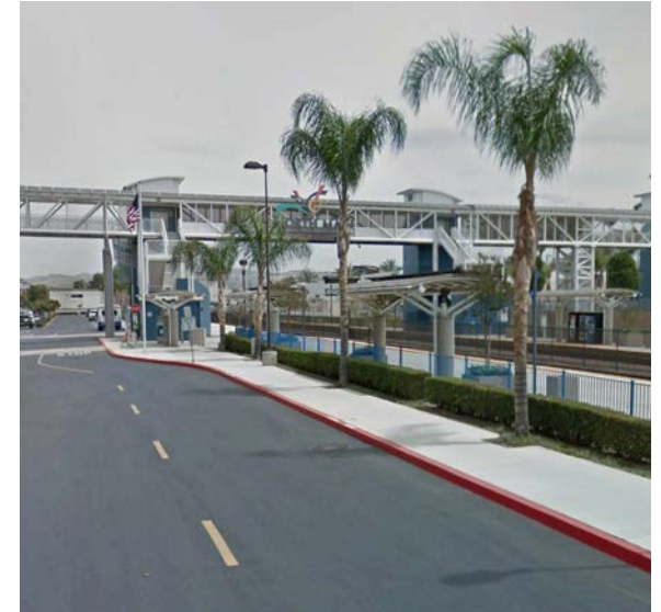
North Main Metrolink Station
