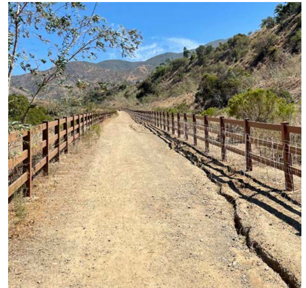
Fencing along the Fresno Canyon Trail
