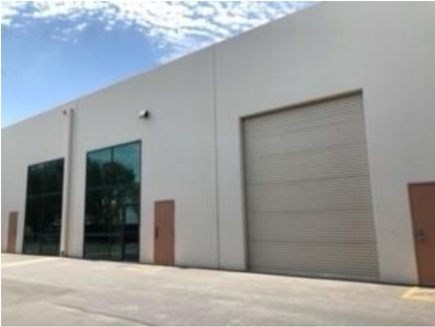
Northeast Elevation (Rear Elevation)
