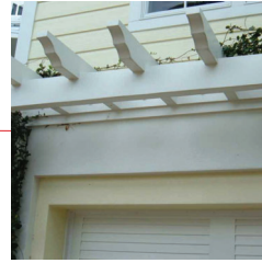
◇ 3X6 HOPE PLASTIC LUMBER TRELLIS BY TANGENT FACTORY FINISH DARK BROWN
