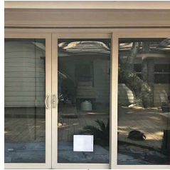
◇ RECESSED VINYL EXTERIOR DOORS & WINDOWS JELD-WEN V-2500 SERIES, BONE COLOR
