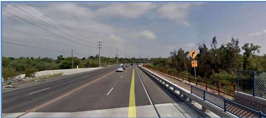
Figure 3-3 River Road Looking Northerly from Bridge
