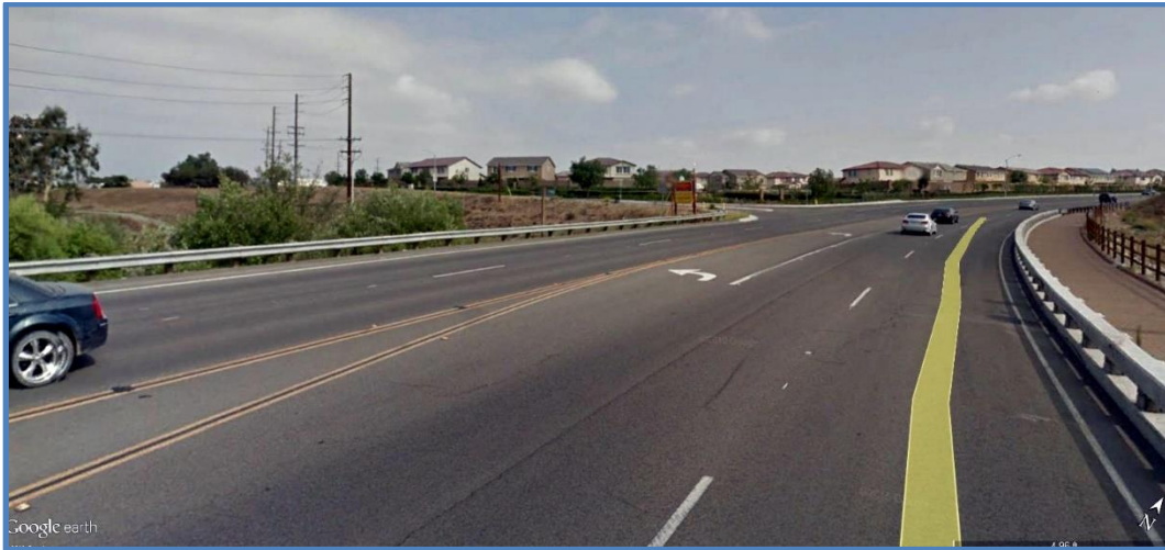
Figure 3-4 River Road Looking Northerly at Baron Drive Intersection
