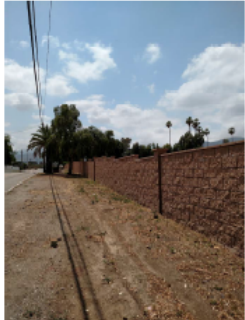
EXISTING 6' HT. CMU WALL W/PLASTERS AT STATE ST.
