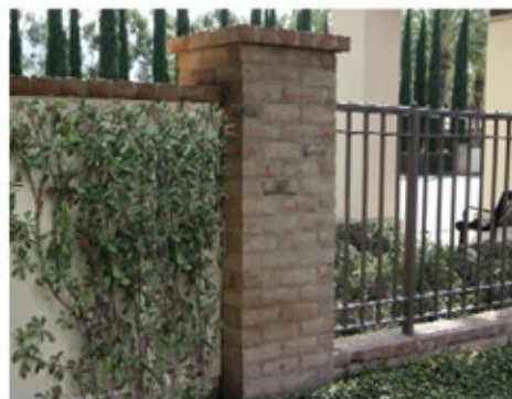
Brick Pilaster
