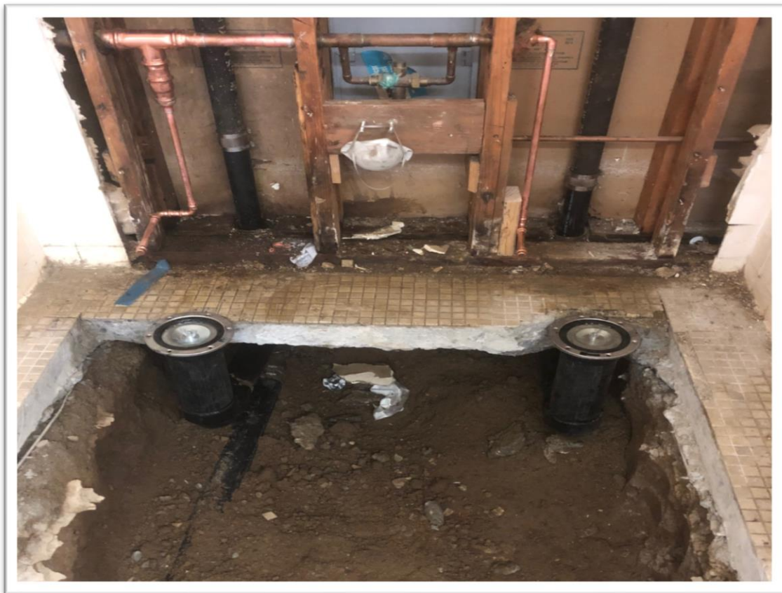
Remove and Replace Corroded Cast Iron Plumbing:
