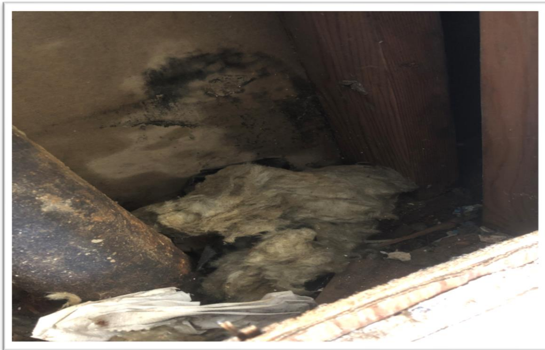
Remove and Replace Corroded Cast Iron Plumbing:
