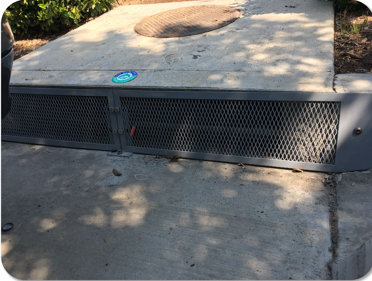
Screen guard BMP for catch basin
