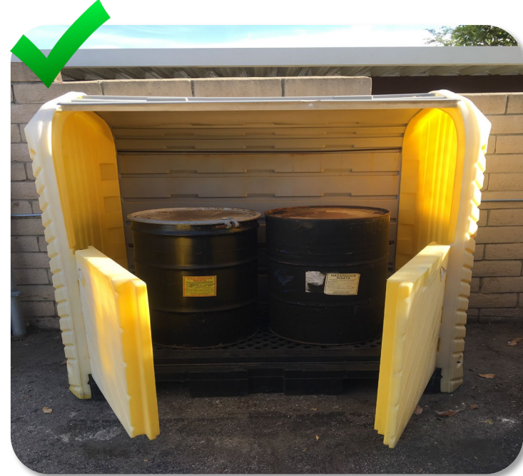
Proper storage containment & cover for materials stored outdoors
