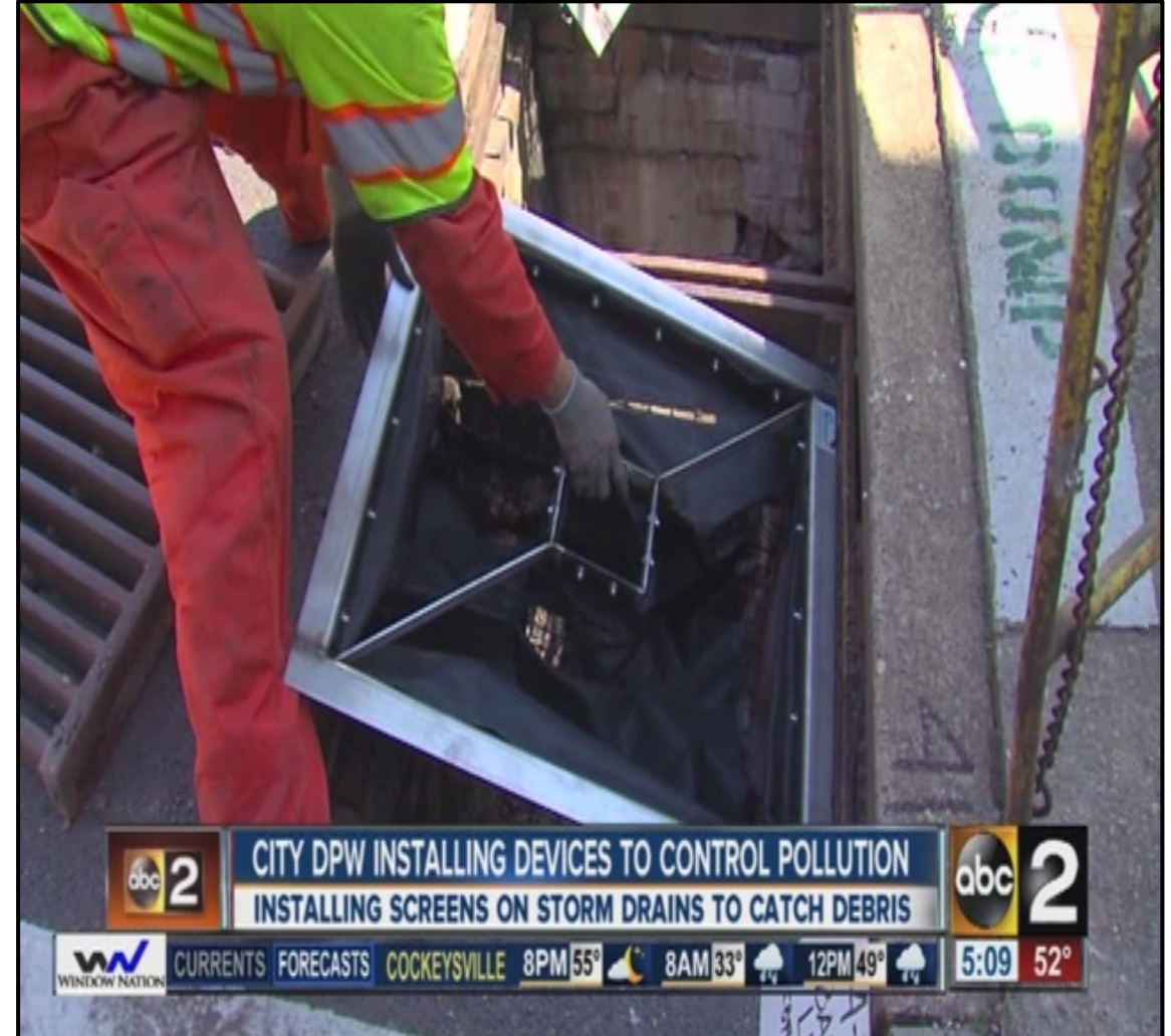
Trash capturing device for catch basin. (Approx. 1,200 to be installed in the City of Corona)
