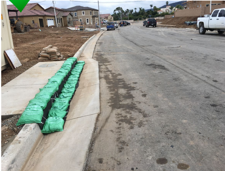
Proper Installation of BMPs for storm drain inlet protection & street sweeping
