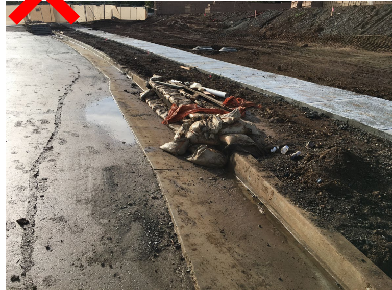
Improper Installation of BMPs
