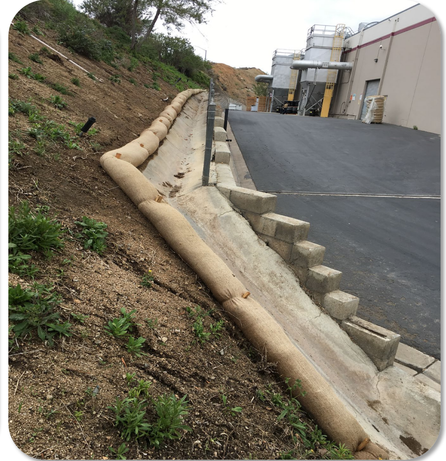
Straw wattle/Fiber roll BMP to prevent sediment discharge
