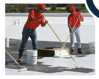
A "cool roof" is a roof with a reflective coating applied that helps reflect heat.
